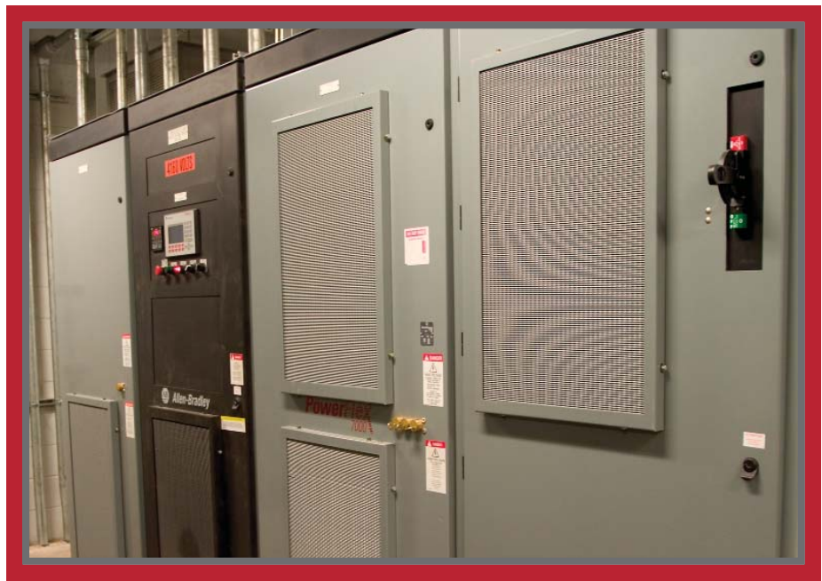
PowerFlex 7000 medium voltage variable speed drives improve process control and help provide maximum efficiency and energy savings.
