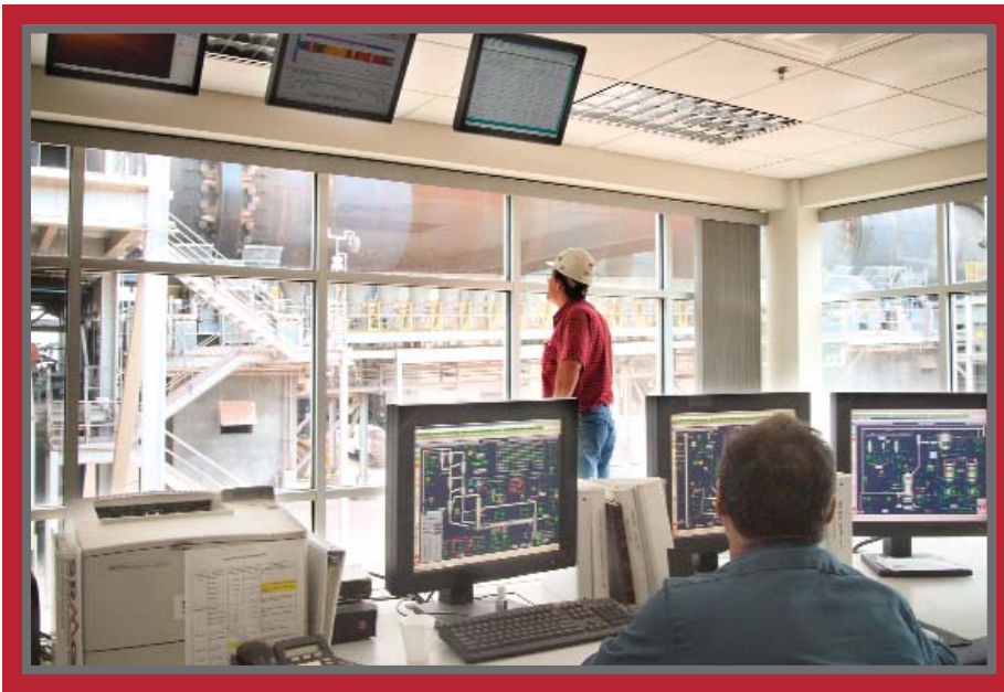
From the Phoenix Cement Company's control room, operators can access plant and production data, and monitor motors using Integrated Architecture technology from Rockwell Automation.
